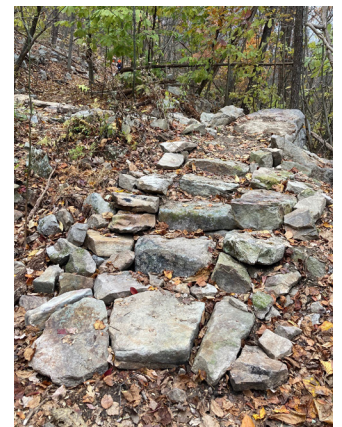
Trail improvements installed by members of the Susquehanna Appalachian Trail Club include rock steps where erosion was problematic.
