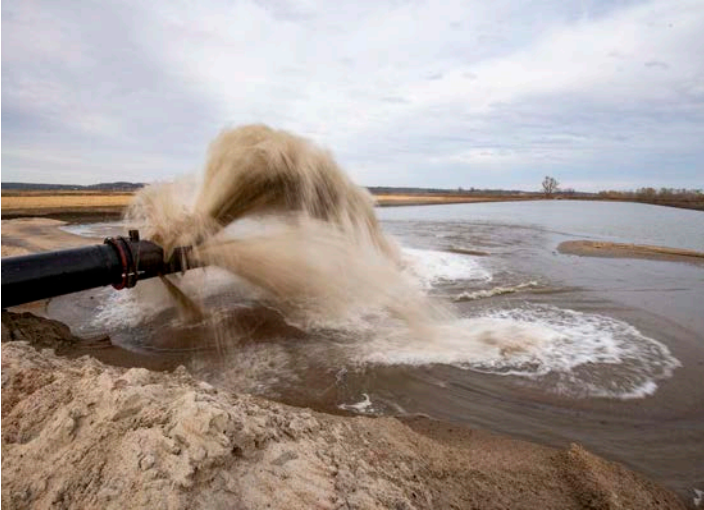
Dredging work along the Missouri River, October 2020.
