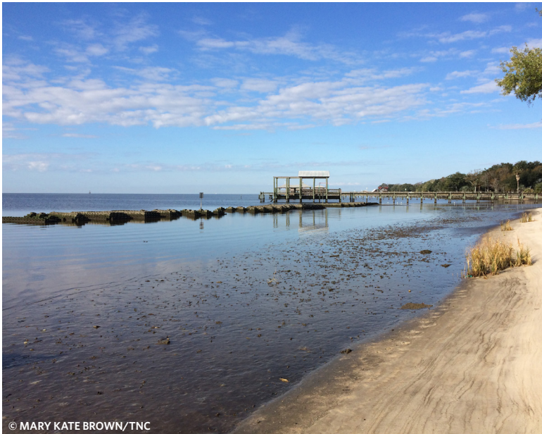
Reef structure helps accumulate sediment.
