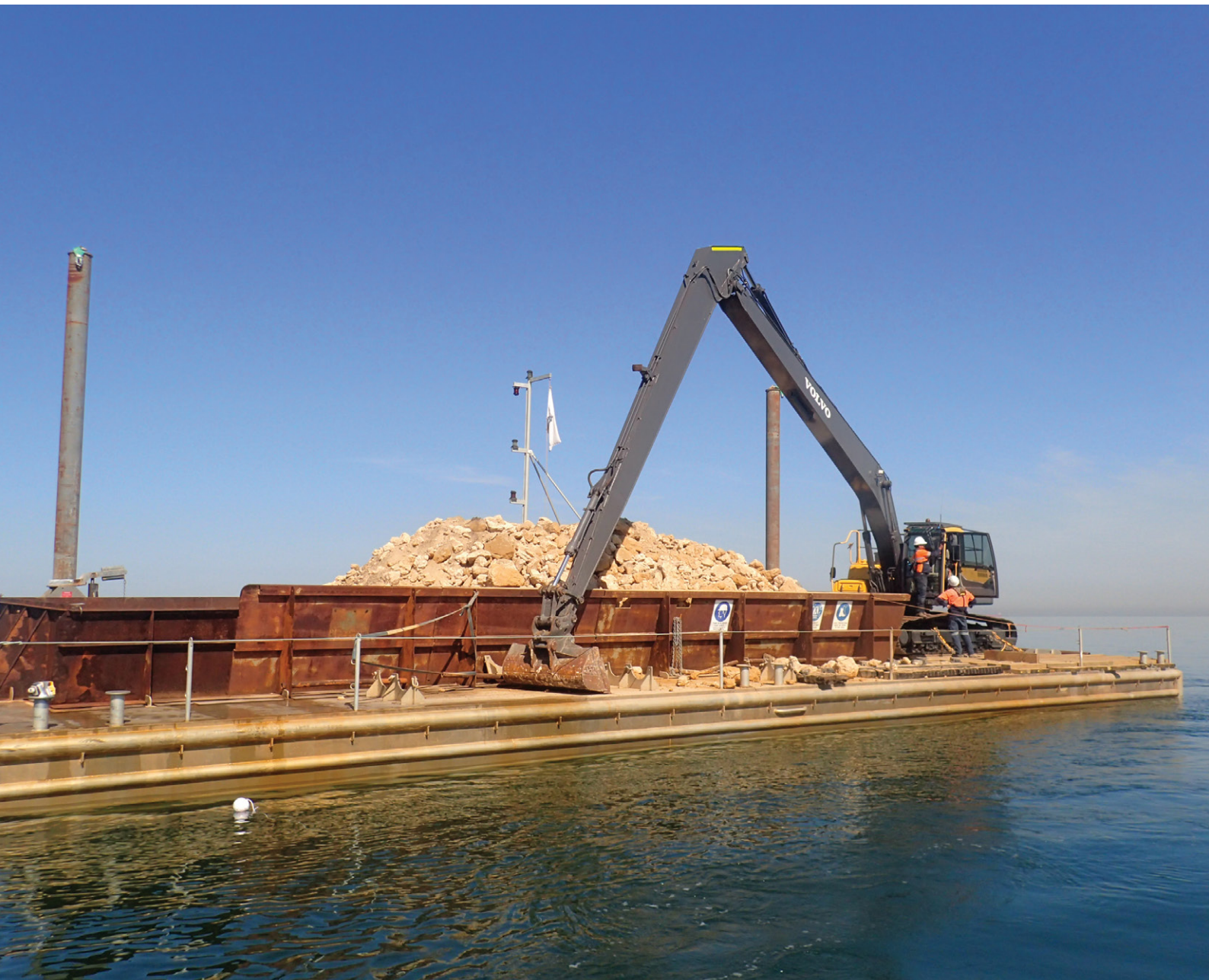
Figure 6.2: Shellfish reef construction at Margaret’s Reef, Port Phillip Bay. Photo: Anita Nedosyko.
