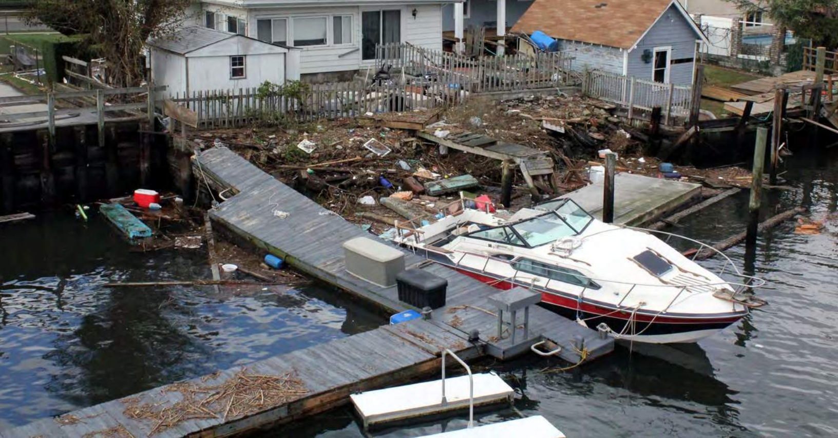
Howard Beach pier and boat damage © Pam Andrade/Flickr via a Creative Commons license
